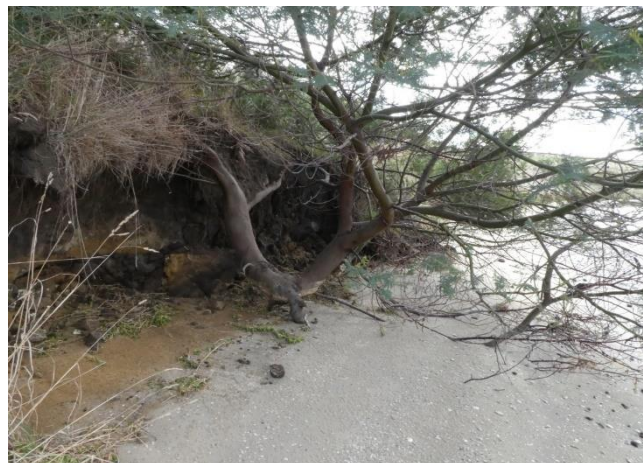
Collapsed wattle on the foreshore
